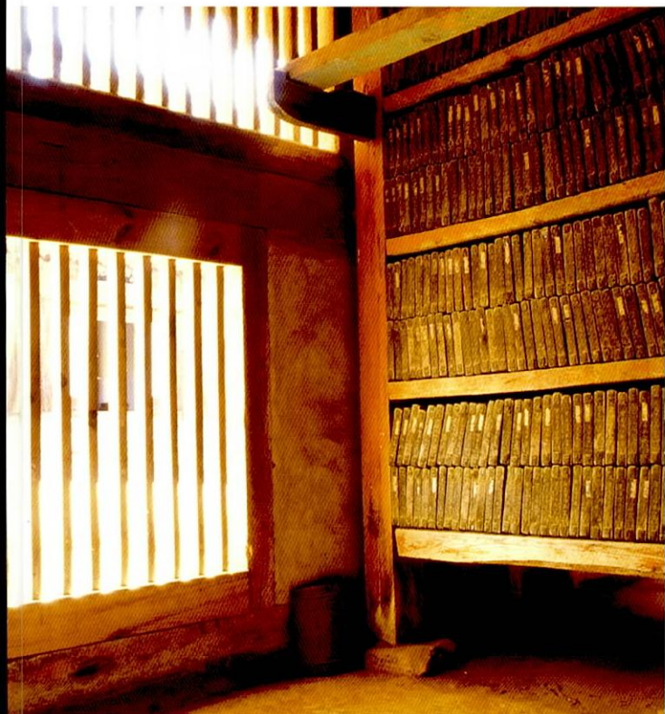
▼ Woodblock shelves and the slatted ventilation windows
